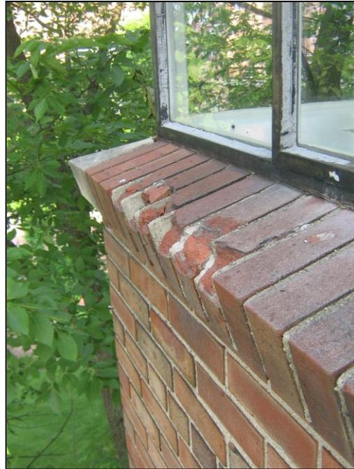
There is one location on the south wall at the top where an area of bricks has shifted. Many of the parapet cap joints are open, and some of the caps have moved or shifted.
