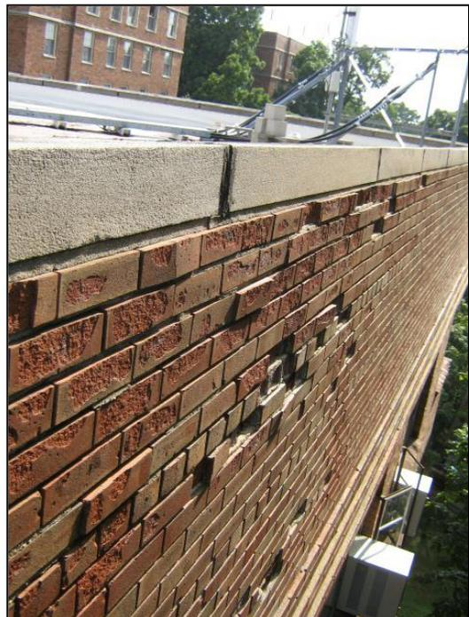
I estimate that there are between 30 and 50 damaged window sills. Some are entirely damaged, while others have only one damaged brick. This is also more prevalent on the south side.
